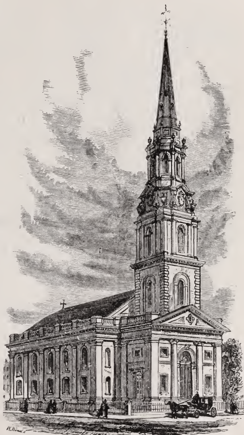
The Arlington-street Church, corner of Boylston Street.
